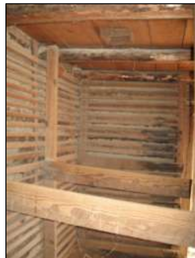
Image 87: The frame potato-curing shed interior retains stove vents and bin racks.
