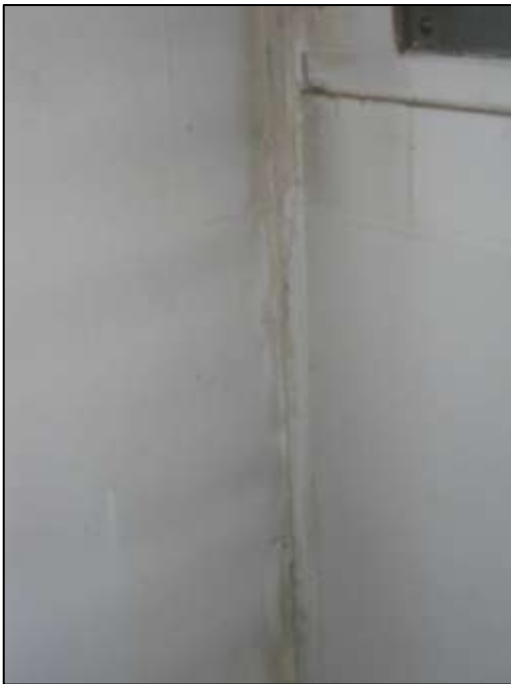
Image 142: Water damage in the infill room interior corresponds to similar exterior water problems.
