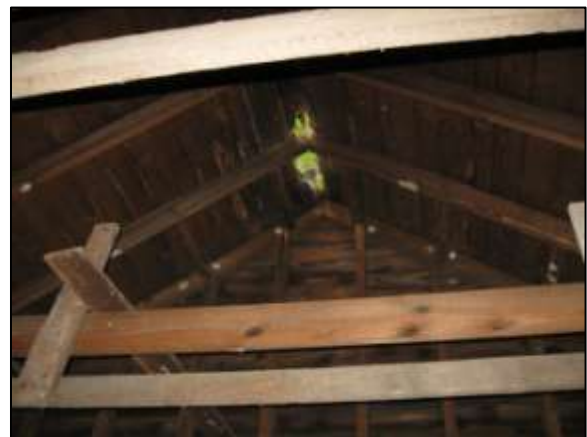
Image 181: Roof damage, now temporarily patched
