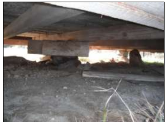
Image 197: The foundation appears to have been repaired and should be assessed.
