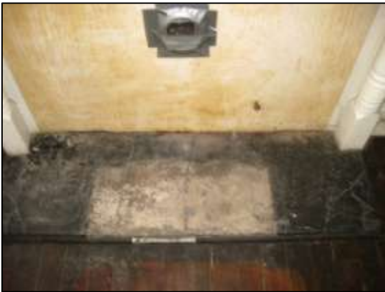
Image 157: Cracked hearthstone in the first floor north room
