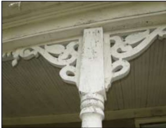
Image 36: The Victorian porch features foliate patterned brackets, drop pendants, and sawtooth drapery.
