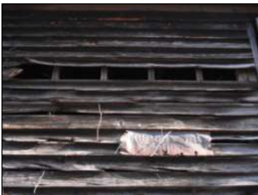
Image 179: Damaged weatherboard
