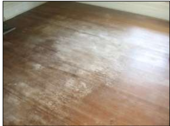
Image 153: Wear and tear on original floor in the south room, first floor
