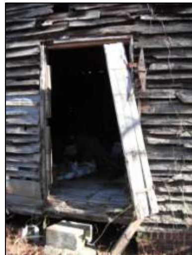
Image 177: The damaged front door fails to protect the building from the elements.
