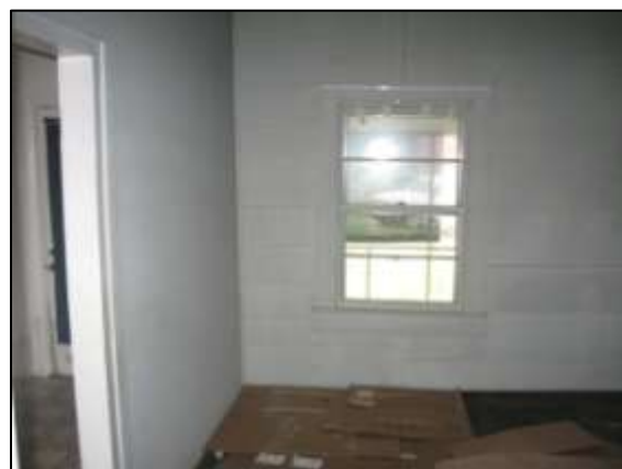
Image 17: The southeast parlor wall is Victorian tongue-and-groove paneling where the original staircase was removed and filled in.
