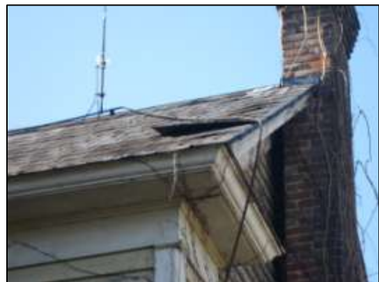
Image 119: There is damage to the roof on the north façade of the Victorian addition
