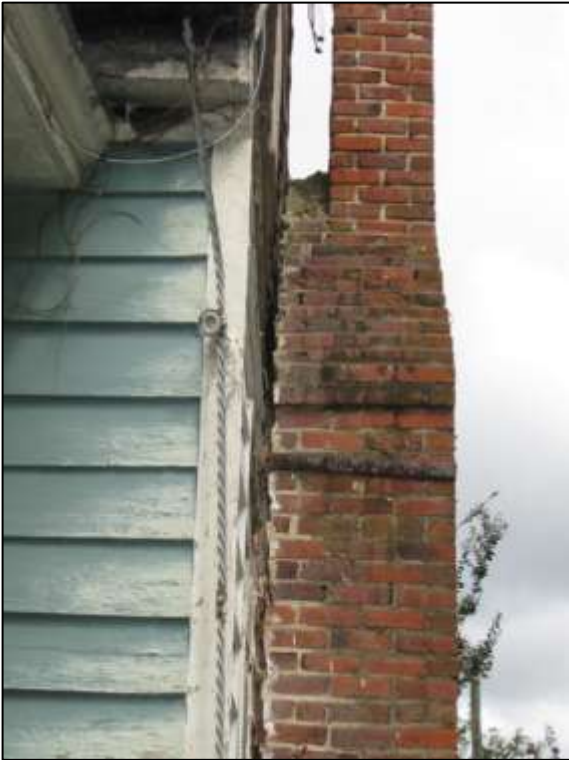
Image 121: The east façade chimney is leaning.
