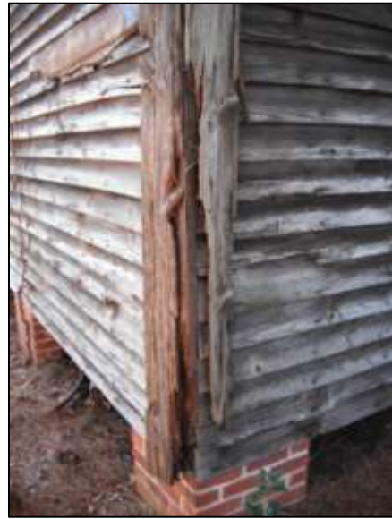
Image 180: Damaged corner boards
