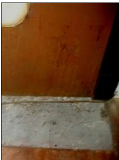
Image 158: Cracked hearthstone in the second floor north room
