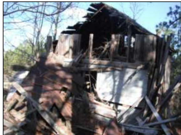
Image 89: The southern section of the tenant house has collapsed.
