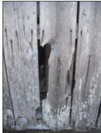
Image 196: The weatherboard on the corn crib is damaged in some places.
