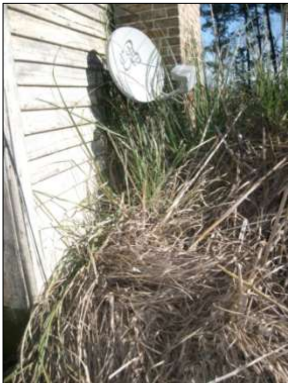
Image 131: Overgrowth of heavy grasses around the foundation on the south façade
