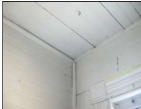
Image 144: Water damage to ceiling and walls in north room, second floor
