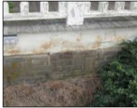
Image 31: The original brick pier foundation is now enclosed.
