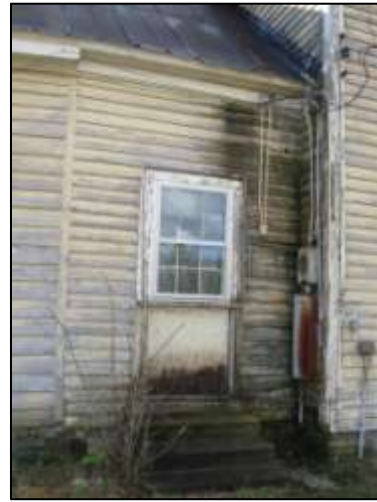
Image 128: There is significant water damage to the north façade of the infill room
