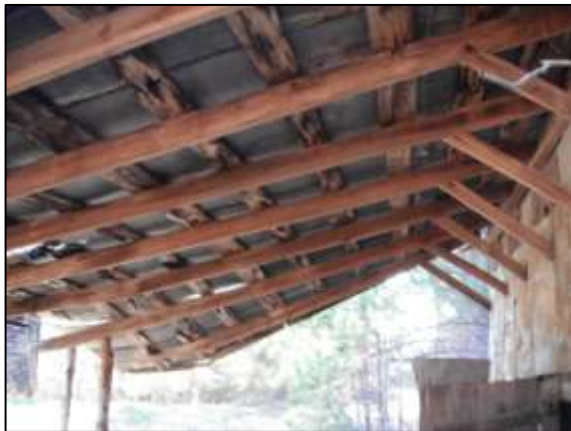
Image 166: Some of the shed roof support beams are in good shape while others need to be replaced.
