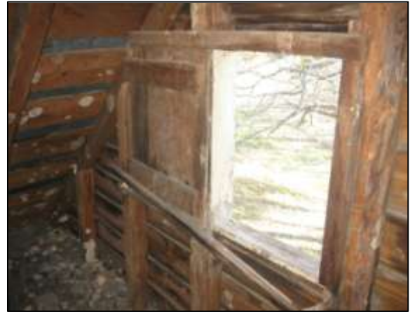
Image 19: Two small windows look east over the shoulders of the chimney and have the original single sash, recessing wood panels.
