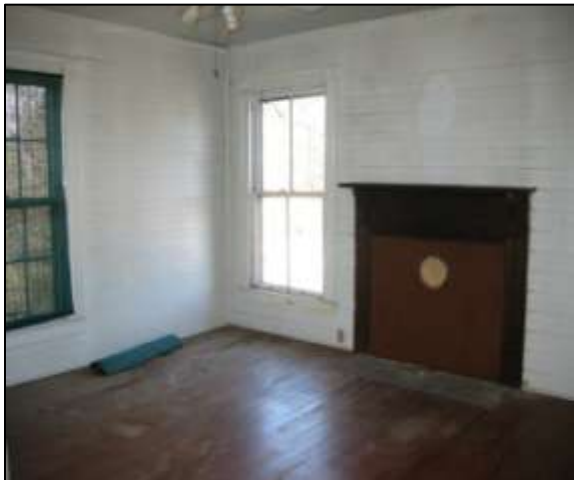
Image 63: The north room on the second floor retains its original tongue-and-groove paneling, pine floorboards, and geometric cornerblocks.
