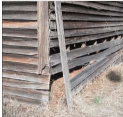
Image 85: The frame potato-curing shed has sawdust insulation.
