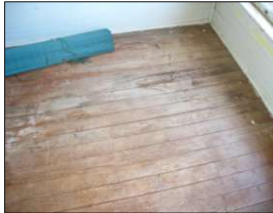
Image 143: Water damage to floor in second floor north room
