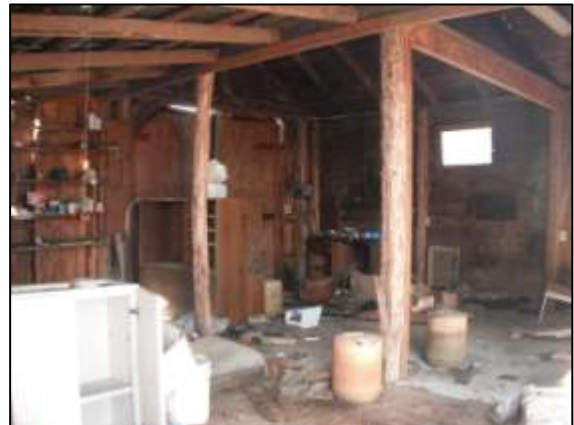
Image 103: The interior of the shed reveals that the north section of the building was the original shed and the south section was enclosed later.
