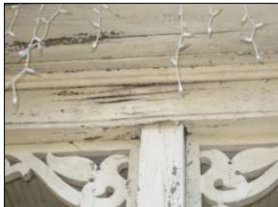
Image 127: Damage to porch roof
