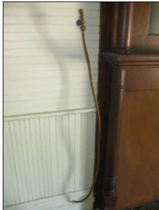
Image 148: Exposed gas line to first floor south room fireplace
