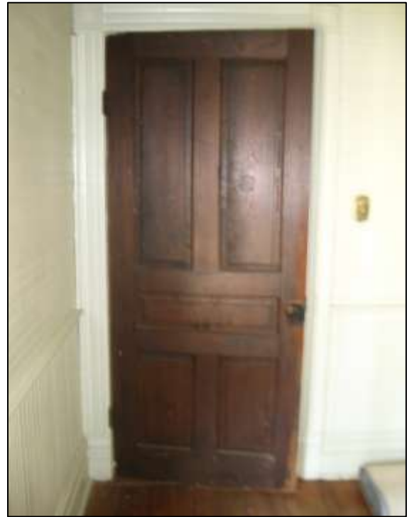
Image 61: The doors are a common five-paneled Victorian design, suggesting they were ordered from catalogs as stock materials.
