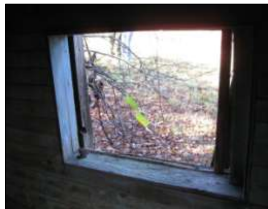
Image 93: The original single sash, recessing glazed windows on the north and west façades.
