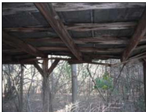
Image 172: Some shed roof support beams are in good condition but others need replaced.
