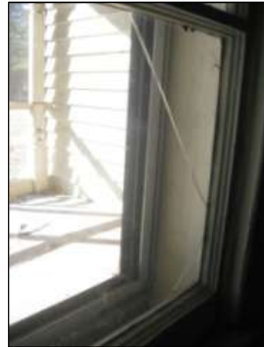
Image 118: There are many cracked or missing window panes, including this one in the parlor.
