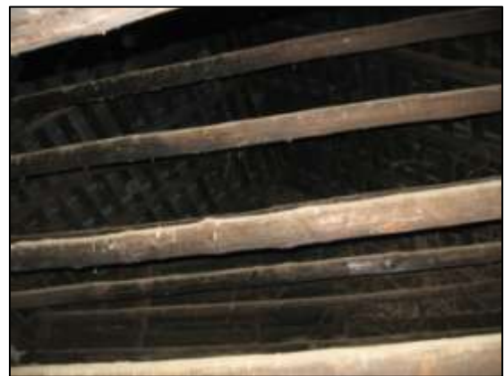
Image 73: The log tobacco-curing barn retains its original pine rafters.
