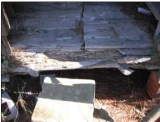
Image 178: The front door sill is damaged
