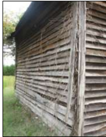
Image 187: The weatherboard on the frame shed is in poor condition.
