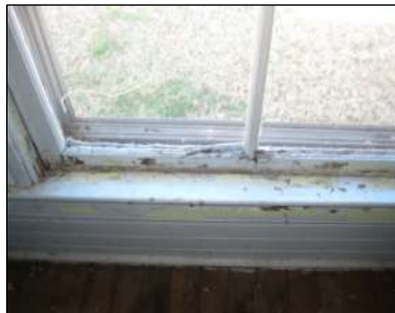
Image 145: Water damage to window in north room, second floor
