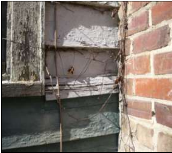
Image 120: The weatherboard is damaged in a few places, including here on the south façade.
