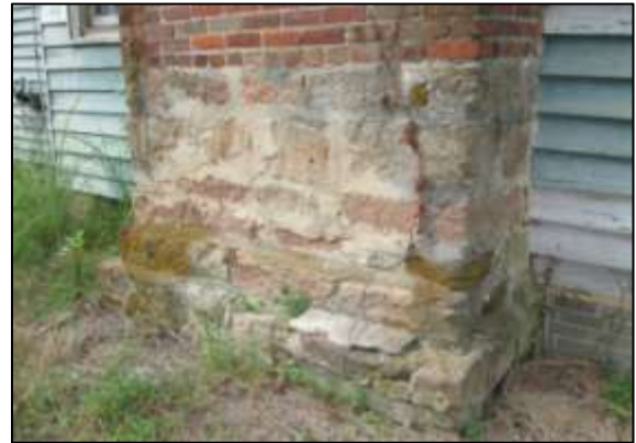
Image 12: There is a roughly coursed stone base on the east exterior end chimney.
