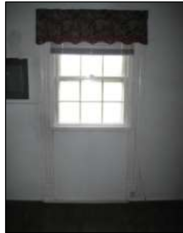
Image 68: The infill room window was originally a door, and the door's ghost marks remain.
