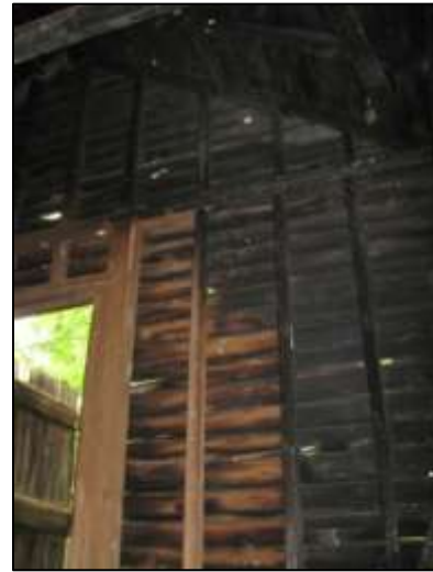
Image 176: Fire damage on the second floor
