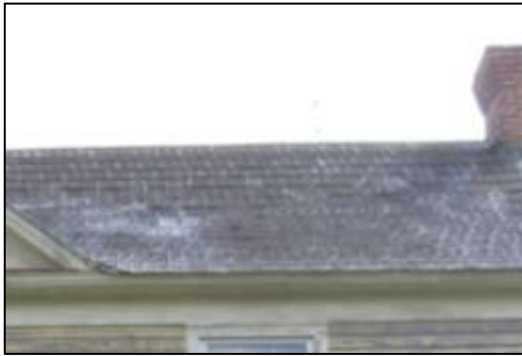
Image 28: The Victorian addition features a decorative stamped-tin roof.
