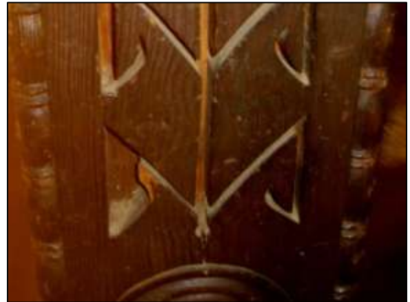
Image 159: Damaged carving on newel post
