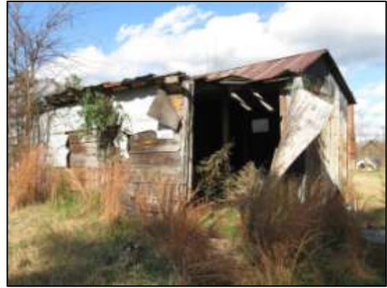
Image 199: The collapsed walls and roof of the shed addition are a threat to public safety.
