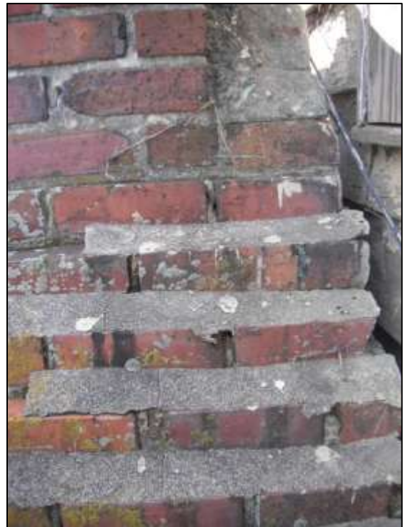
Image 123: Improper repairs to east chimney
