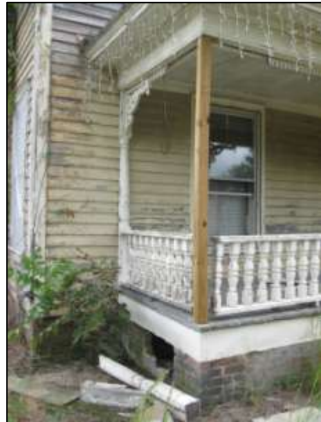
Image 125: One of the original porch posts was replaced and the original is lying in the yard.
