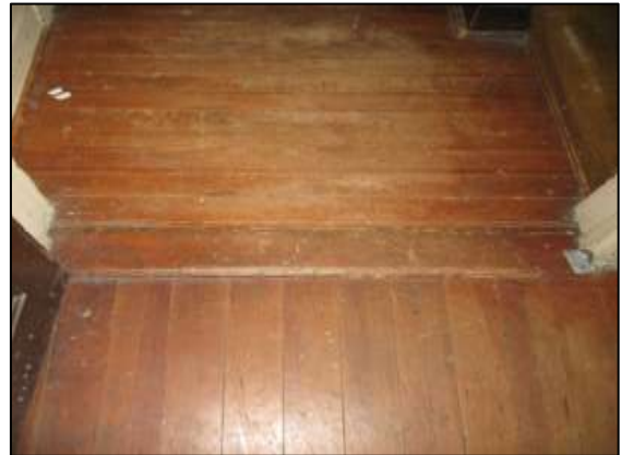
Image 55: The first floor retains its original pine floorboards. (south room and central hall pictured here)
