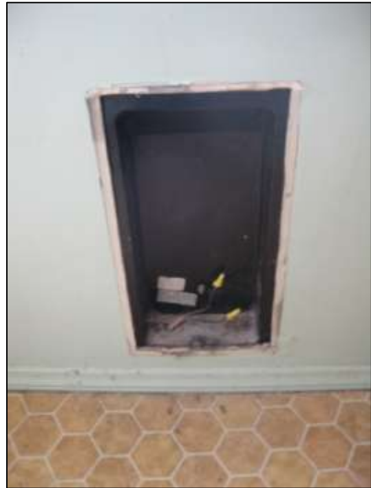
Image 147: Exposed wires in the central hall bathroom
