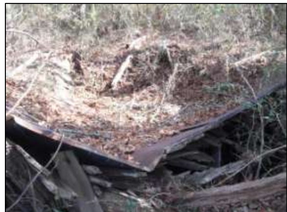
Image 182: Collapsed roof over ordering pit
