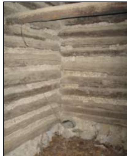
Image 72: The log tobacco-curing barn features clay chinking.
