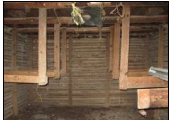
Image 82: The log potato-curing shed interior features stove vents and bin racks.
