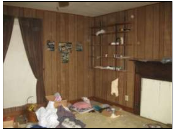
Image 65: The south room has modern paneling over the original tongue-and-groove paneling.
