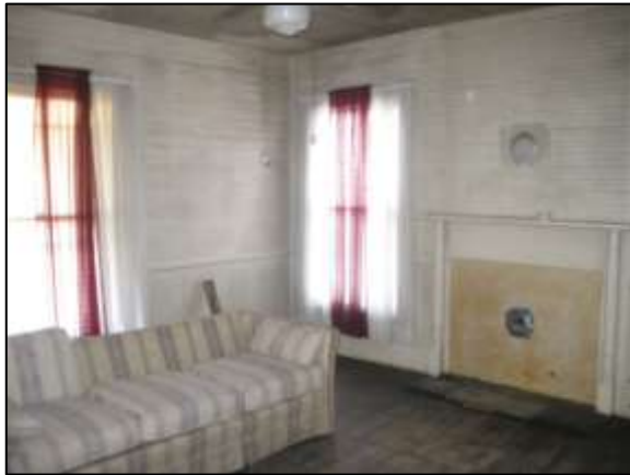
Image 52: The north room, first floor, with the original tongue-and-groove paneling and ceilings and bead board wainscoting below the chair rail.
