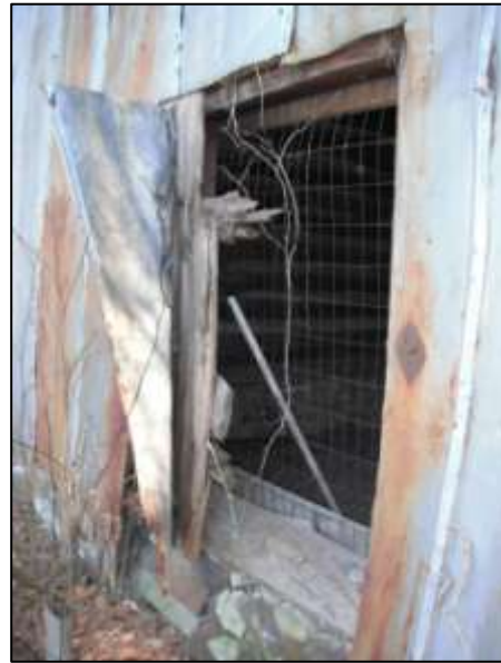
Image 162: Damaged tin cladding
