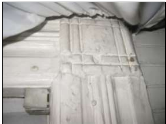
Image 154: Wear and tear on window frame in the north room, first floor
