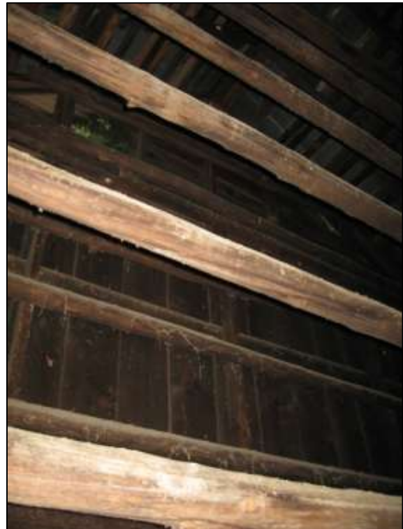
Image 75: The frame tobacco-curing barn retains its original pine rafters.
