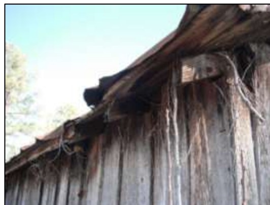
Image 185: The roof on the log shed is damaged
