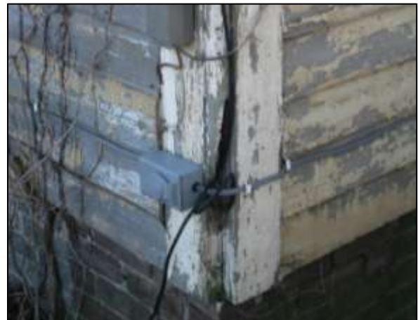
Image 136: Damage to northwest corner board on Victorian addition
