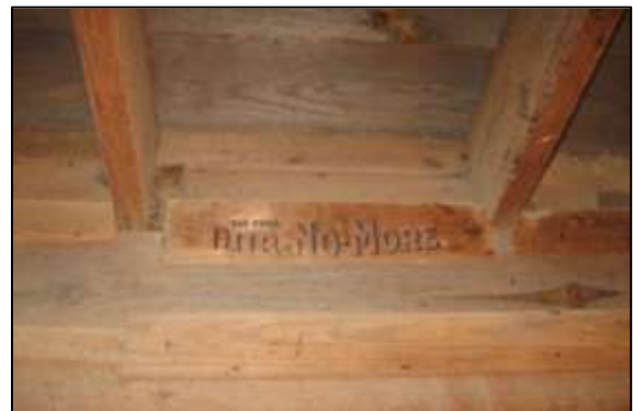
Image 86: The interior of the frame potato-curing shed was repaired using shipping crates.
