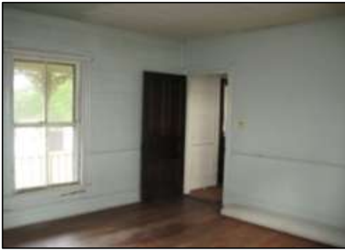
Image 58: The first floor features tongue-and-groove paneling and ceilings, as well as beadboard wainscoting. (south room here)
