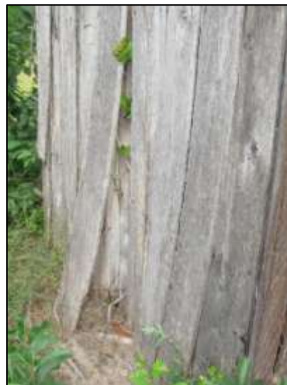
Image 184: The weatherboard on the log shed is damaged in several places.
