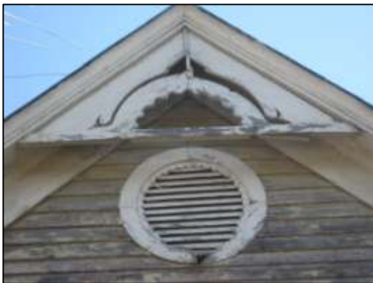
Image 124: Damage to center gable millwork and missing spindles
