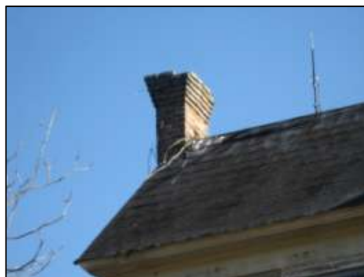
Image 133: Roof damage caused by overgrowth on north chimney
