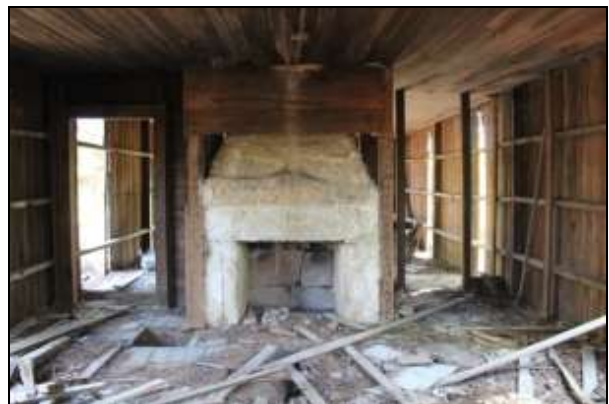
South Room. Note the roughly parged stone chimney and remains of the stack enclosure.
