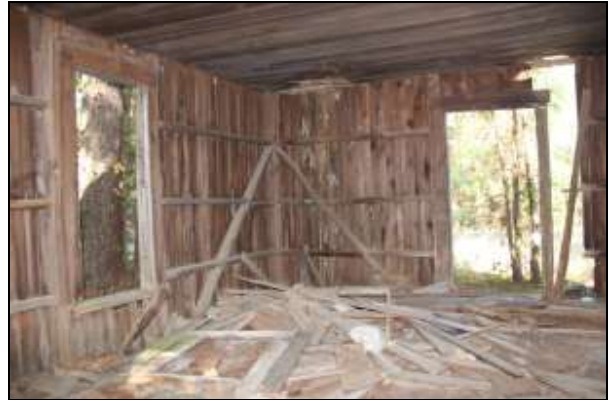
North Room. Note the corner braces and lack of interior finishing.
