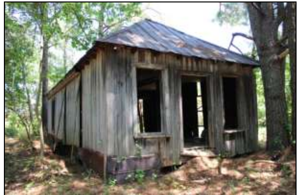
Southwest elevation. Note the barn tin roof and tin-wrapped foundation.
