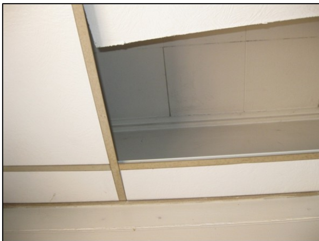
The original sheathing on the hall ceiling is covered by a late-twentieth-century tile ceiling and a modern drop ceiling
