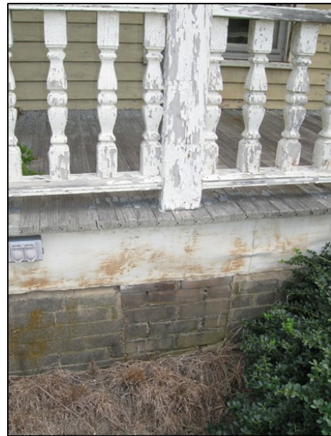
Brick Pier Foundation
