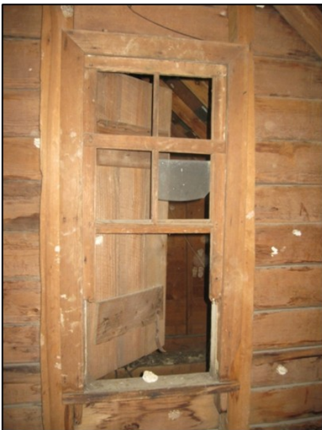
There is also the original window facing Creedmoor Road on the west façade, now not visible behind the addition. This window was four-over-four glazed with a double hung sash and retains the original shutter.
