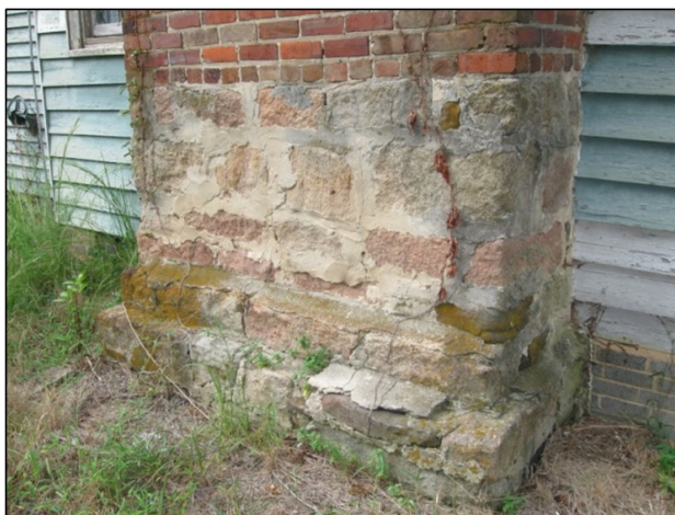
There is a very roughly coursed stone base on the exterior end chimney on the east façade
