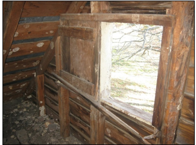
Two small windows look east over the shoulders of the chimney and have the original single sash, recessing wood panels. These windows are now the only access to the loft
