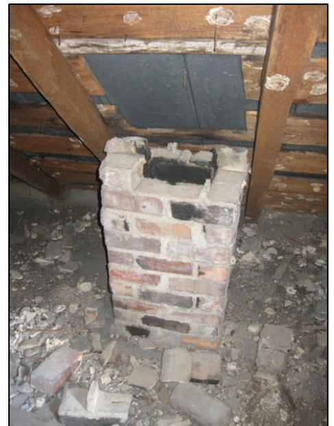
There is a stove flue in the northeast corner of the loft, possibly from the later addition of a stove in the hall
