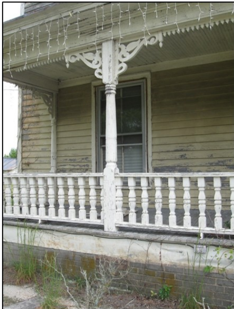
The Victorian porch features delicate millwork that may have been partly ordered from popular catalogs and partly designed and carved by a local builder
