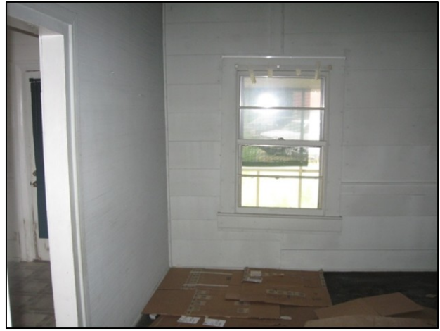
The southeast parlor wall is Victorian tongue-and-groove paneling where the original staircase was removed and a wall constructed around the turn of the century
