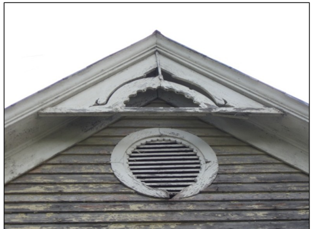
The center gable of the west façade features a louver window and decorative millwork bracket
