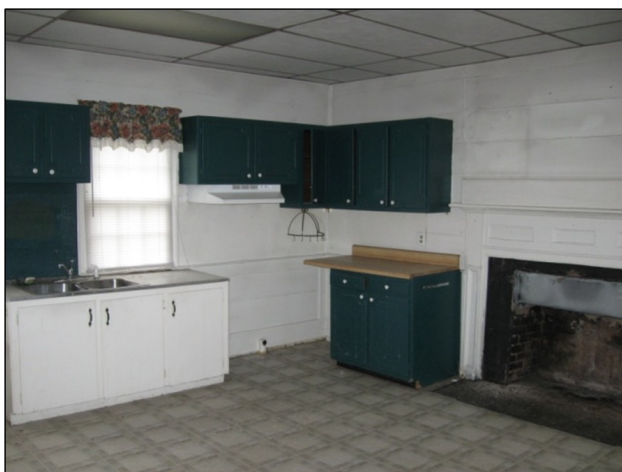
The original hall has been altered with the addition of modern kitchen features, but retains its original architecture. The original ceiling sheathing is covered by a modern drop ceiling, and the linoleum flooring was installed on top of the original pine
