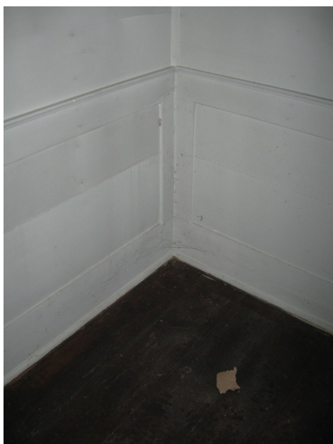
The wood paneling in both the hall and the parlor is original and features flush-sheathed wainscoting, and the original pine floor is still visible in the parlor
