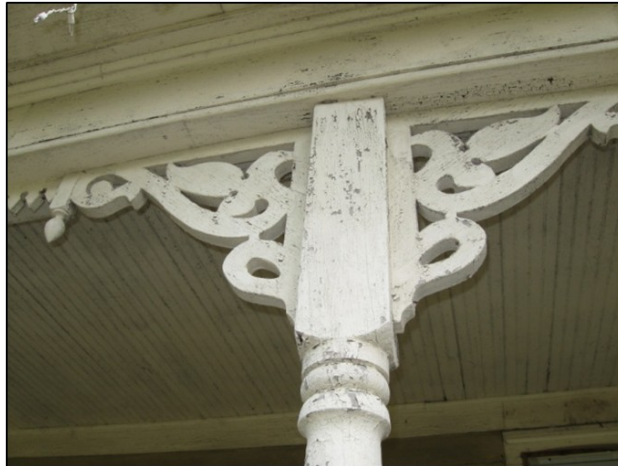
The Victorian porch features foliate patterned brackets, drop pendants, and sawtooth drapery
