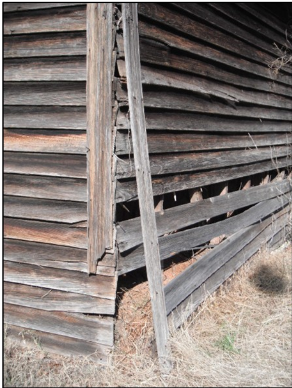
Frame Potato-Curing Shed, Sawdust Insulation
