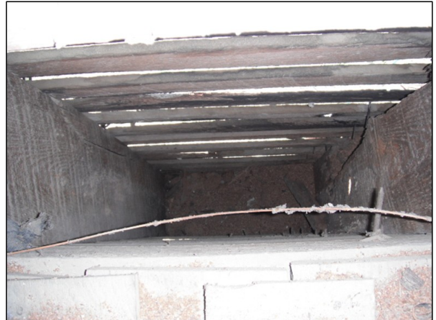
Frame Potato-Curing Shed, Sawdust Insulation
