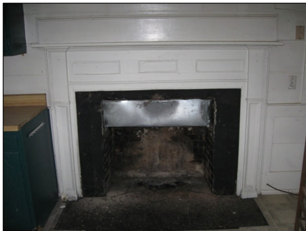
The transitional Federal-Greek Revival style of the hall-parlor house is exemplified in the hall mantle, which features recessed panel frieze and recessed panel pilasters
