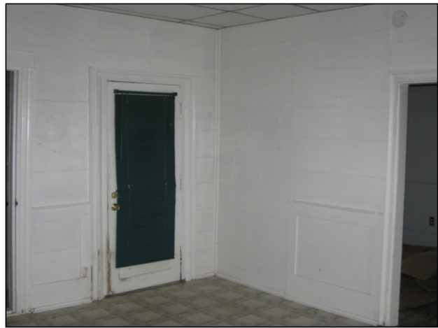
The staircase to the second floor sleeping loft was originally accessed by a staircase leading from the hall through the parlor to the second floor, which was removed and the wall was filled in with tongue-and-groove paneling
