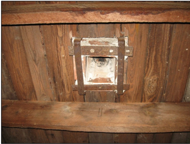
Frame Potato-Curing Shed Central Flue
