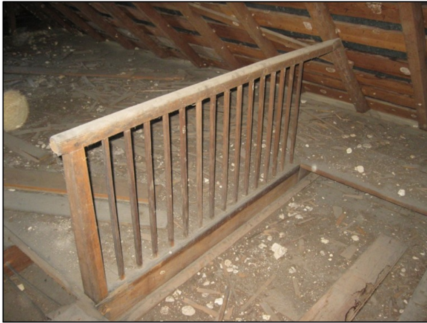
The original balustrade for the loft staircase is intact on the second floor
